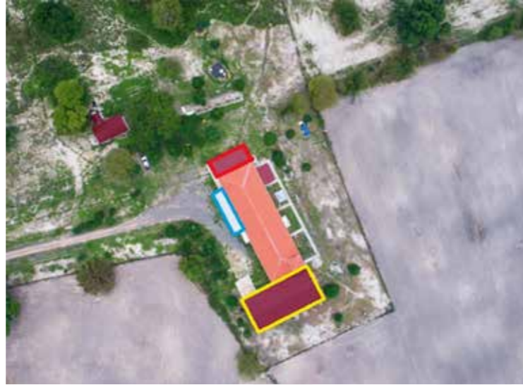
The slaughterhouse and meat processing plant in Namxuang. Development works indicated with colours: Yellow – holding pens; Red – packaging room; Blue – cold storage rooms
