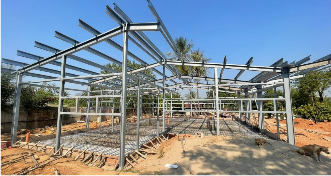
The steel structure of the building of the processing plant
